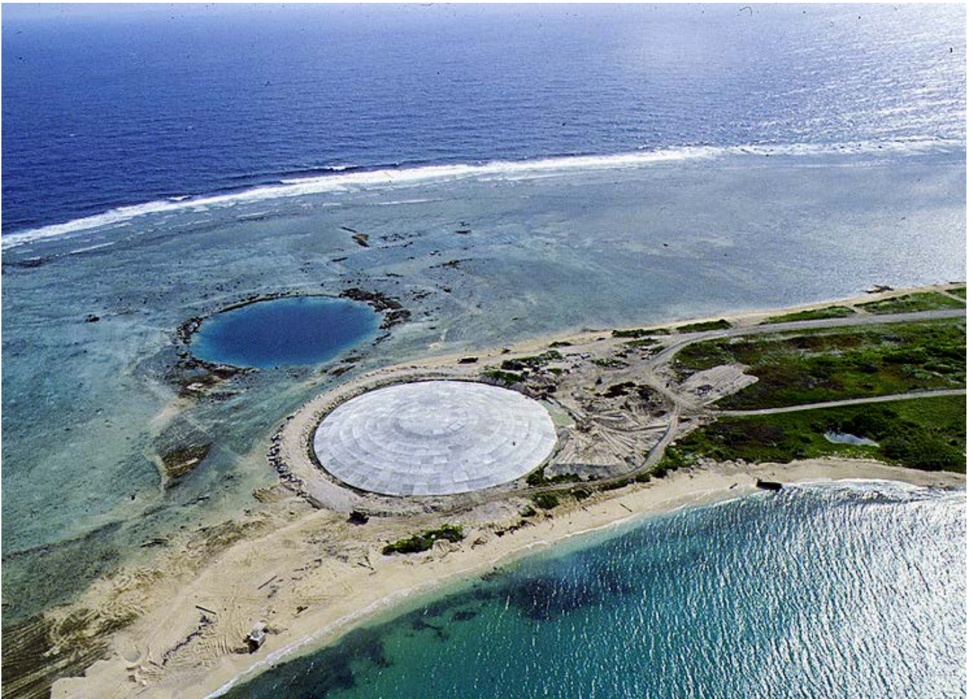
The Runit Dome: On the island Runit, one of about 40 islands of the Eniwetok atoll, a nuclear weapons test formed a crater with a diameter of more than 100 m. The crater was later filled with more than 100 000 cubic meters of plutonium-containing soil from other parts of the atoll and covered with a cement dome.
